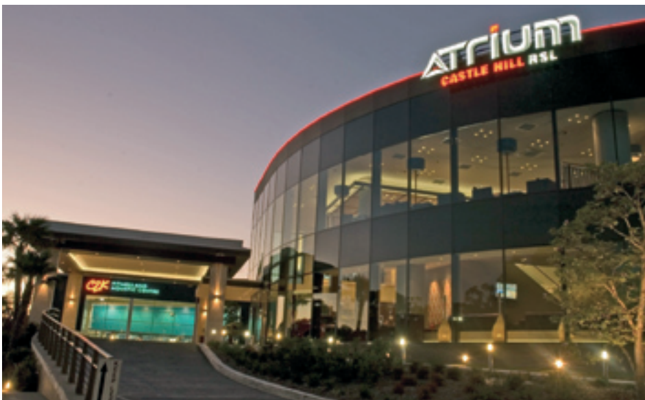
Castle Hill RSL saved $500,000 on their roof restoration!
